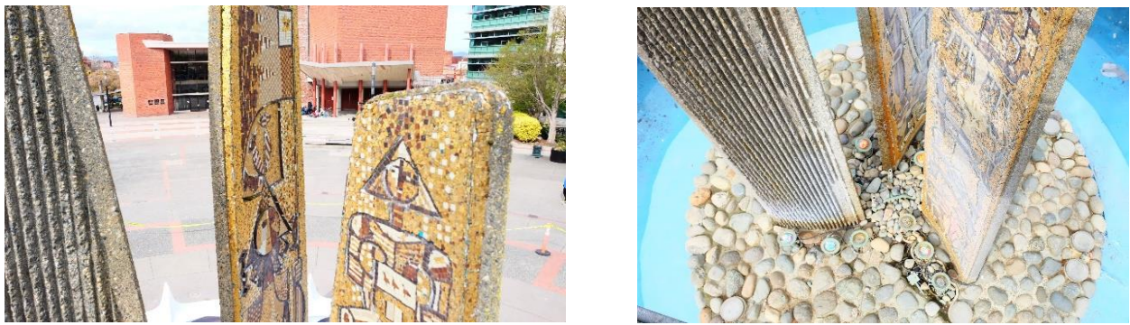
Upper surface conditions on left with moss/lichens. base levels of surface with whitish film.
